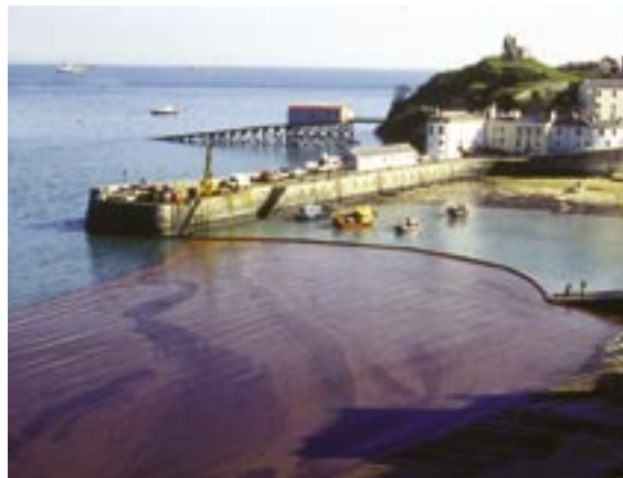
Expenditure and loss of revenue: closing off a port using a containment boom
