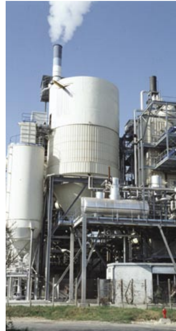
Specific treatment plant for industrial waste, Gironde, France
